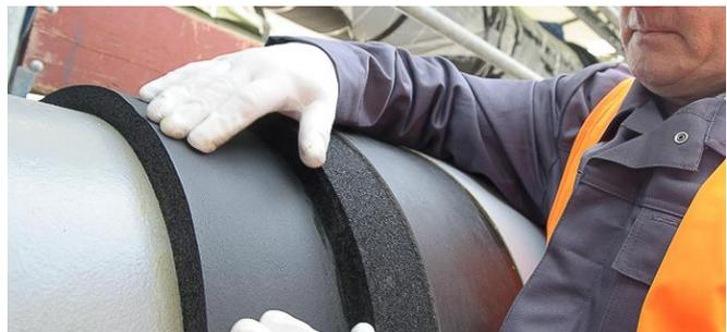
Figure 1: Mineral wool acoustic insulation system (A) & flexible plastic open foam acoustic insulation system (B)
